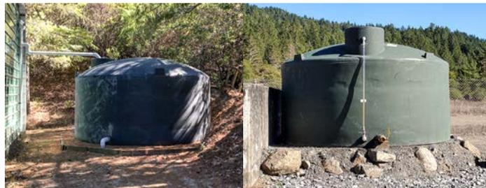
The two newest water tanks in the Annapolis area. One is filled from a roof catchment system, the other will have a catchment system added this winter.
